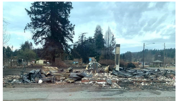
What's left of a home in Gates, Oregon
